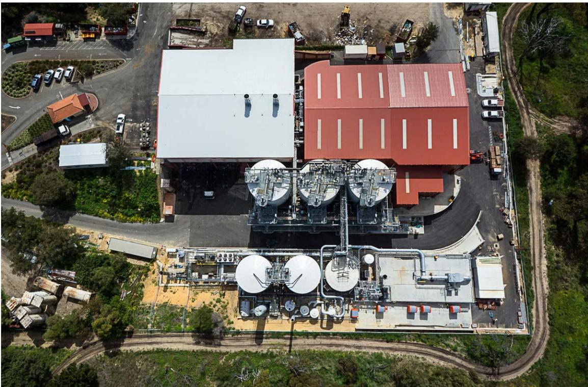
**Figure 2:** Aerial view of the AnaeCo™ AWT Plant showing the existing WMRC transfer station, AnaeCo™ Materials Recovery Facility, DiCOM™ Bioconversion Facility, process water tanks, odour management system and power generation system.
