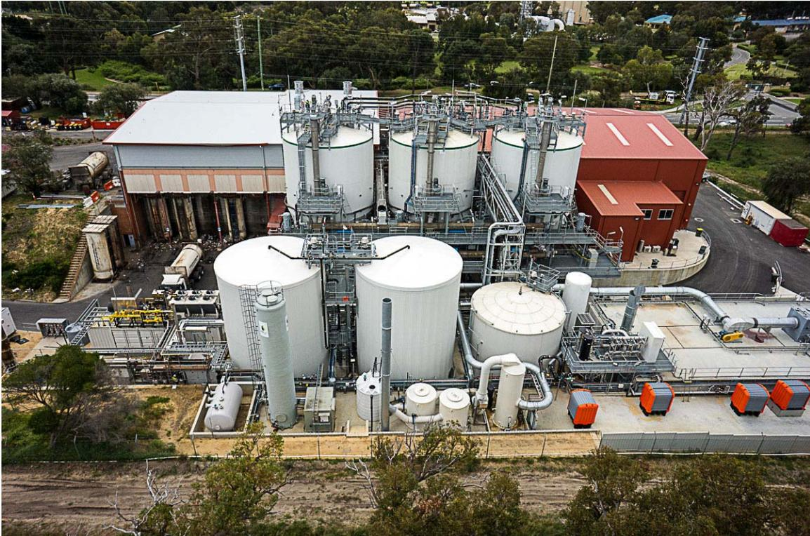
**Figure 3:** The AnaeCo™ Bioconversion Facility (BCF), marked by the 3 large vessels in the background, will digest and compost the organic fraction of MSW using the DiCOM™ process over a period of 21 days - resulting in the production of biogas and stabilised organic fertiliser.
